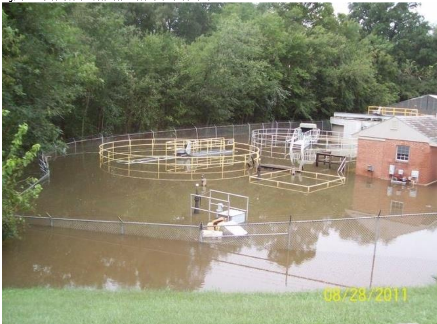
Figure 4-4: Greensboro Wastewater Treatment Plant 8/28/2011
